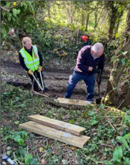
Installing the new steps to make the path easier to walk.
