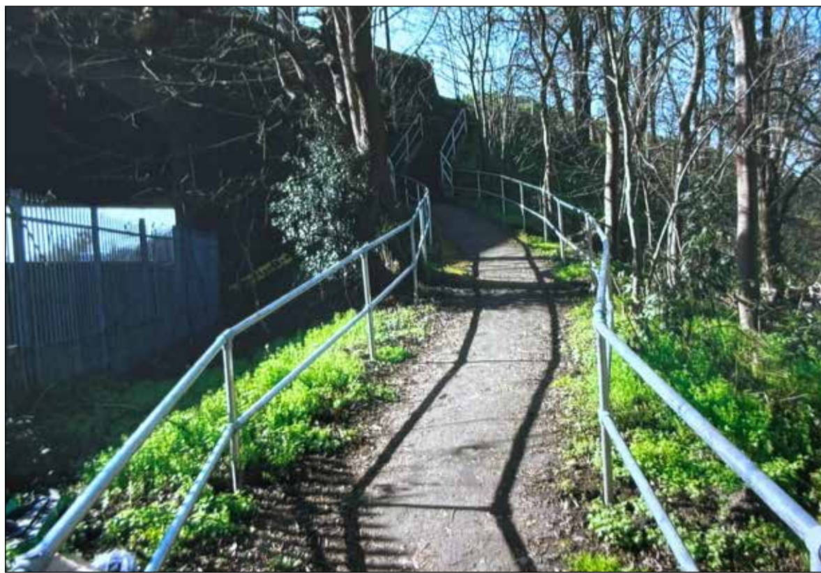
The new handrails on steps near Hall Place in Bexley
