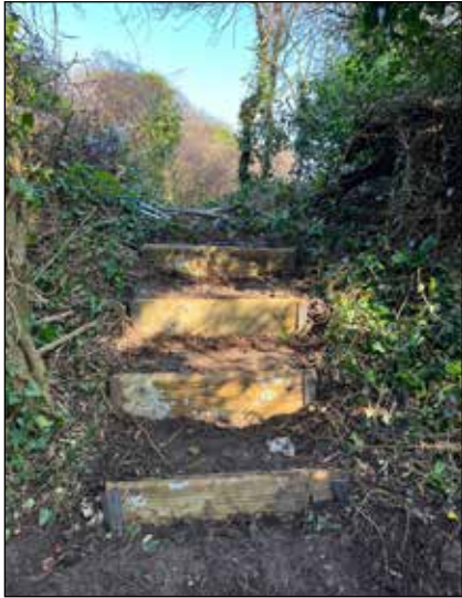
The steps in place.
