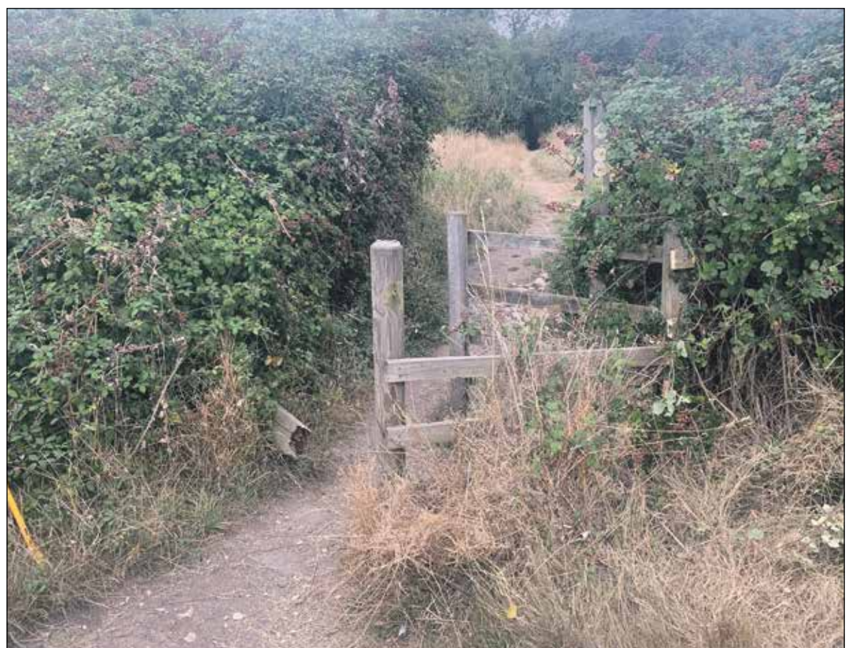
A dilapidated timber kissing gate prior to removal and replacement with a steel pedestrian gate.
