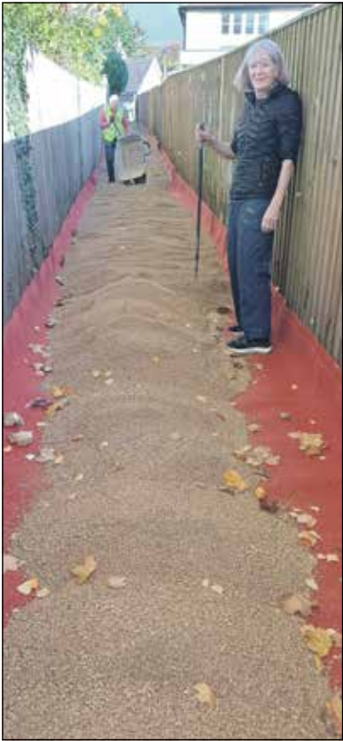
Dumping and spreading gravel over the newly-laid tennis carpet. Photo: Bob Merry
