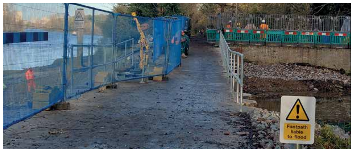
The repaired section of the Thames Path between Richmond Lock and Kew.
