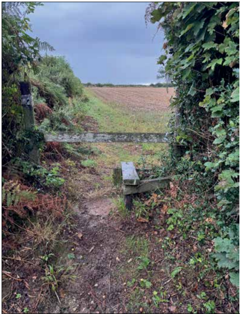
One of the stiles ready to be replaced at Tincleton, Dorset.
