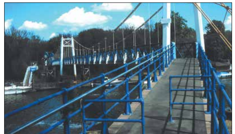
Repairs to the suspension footbridge main structure and lock cut iron truss footbridge at Teddington Lock have been completed.
