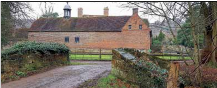
The bridge from the south.
