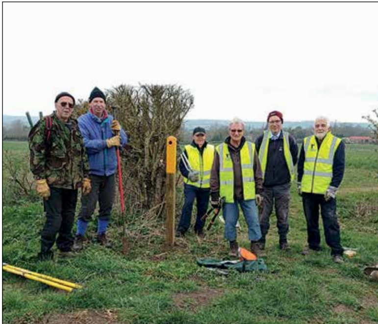
Installing the final marker post at Bletsoe. Photo: Barry Ingram
