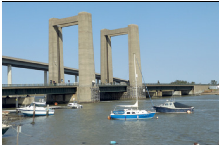
The Kingsferry Bridge, gateway to Sheppey. Photos: Robert Peel.
