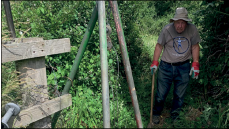
Phil Dudley was relieved that the base of the timber post had finally been lifted clear using the group's makeshift tripod and winch.
