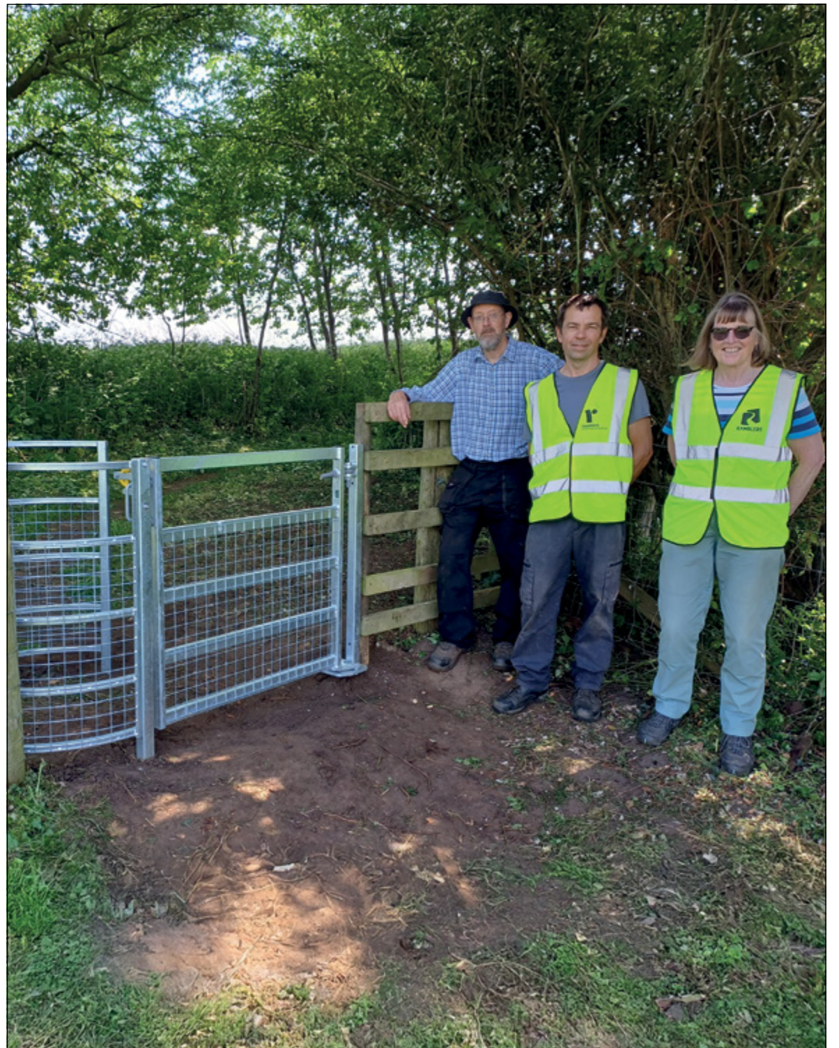
Three members of Thame & Wheatley group's path maintenance team after replacing a stile with a Berkswell kissing gate on the Oxfordshire Way in Stadhampton. Photo: Bob Merry
