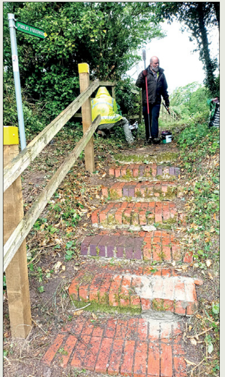
Bedfordshire's very active RIPPLE team recently worked at Billington to clear this path and install new handrails. Photo: Barry Ingram.
