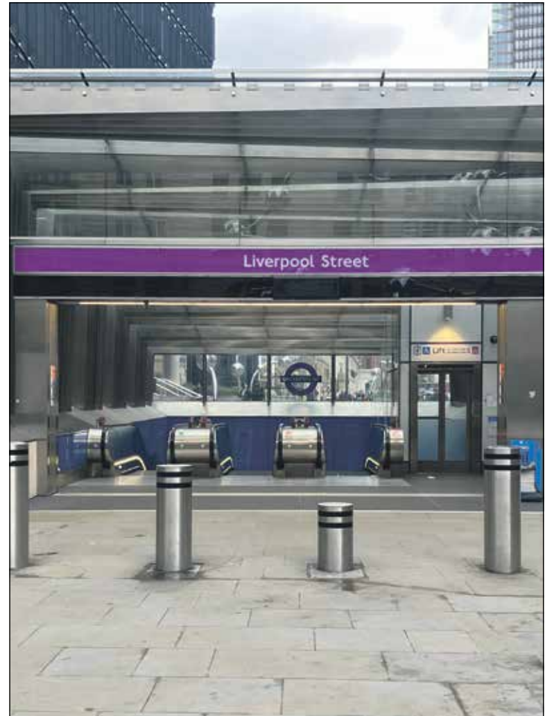
The entrance at Liverpool Street with lift adjacent.
