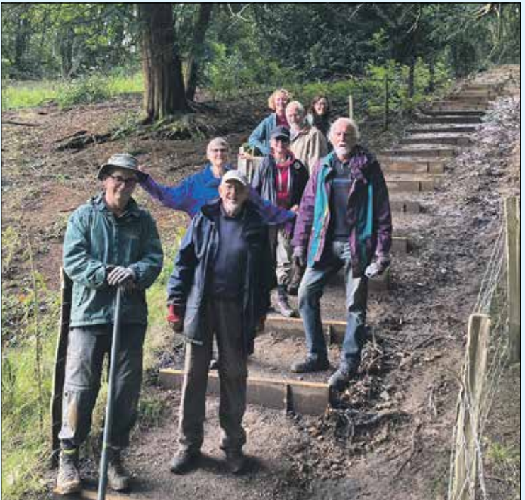
At work on the steps at the Wotton Estate. Photo: Thomas Chatfield/SCC
