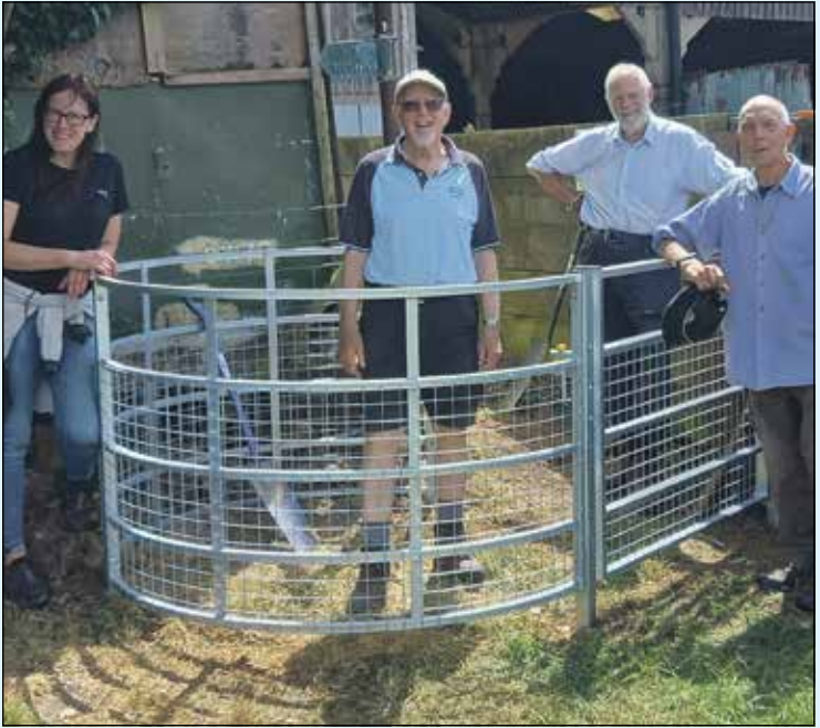
One of two gates installed at Dogkennel Green. Photo: Pauline Butcher
