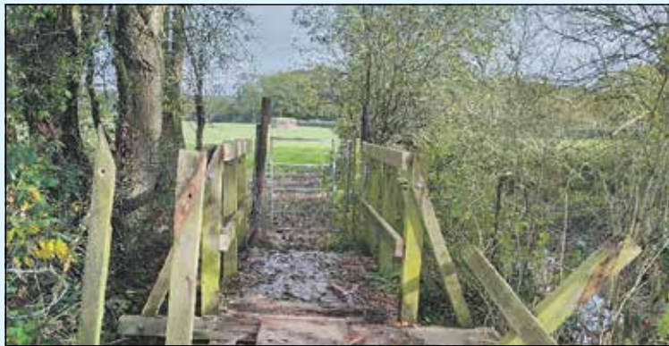
The original footbridge during disassembly.
