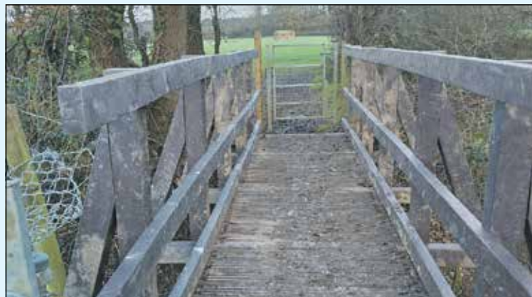
The finished replacement (although somewhat muddy) footbridge.
