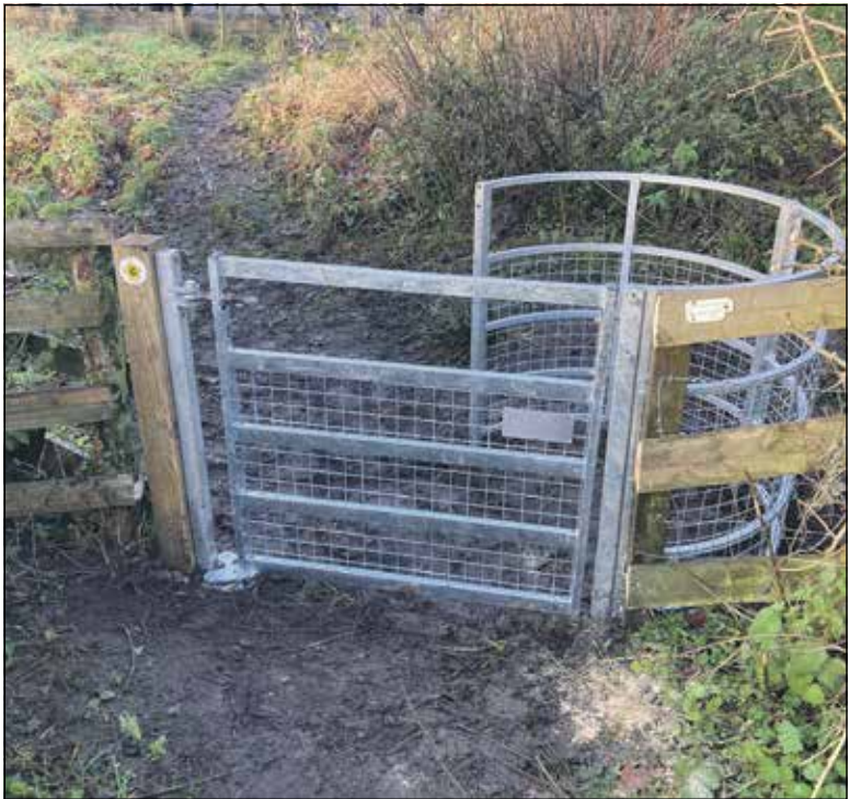
The new gate in Whitchurch. Photos: Bill Piers.
