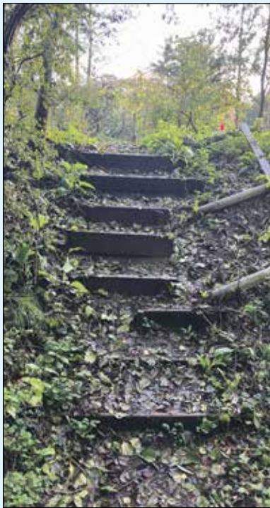
The steps on the west side of the road before the work.
