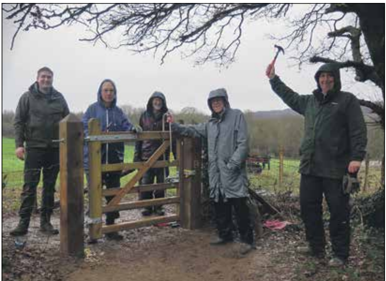
The gate is installed.
