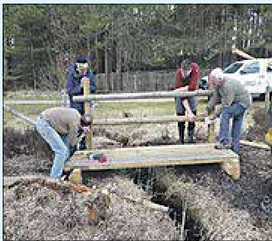
A footbridge is installed.
