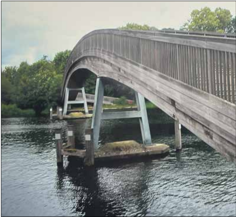
The Temple Footbridge (grid ref SU 835843).
