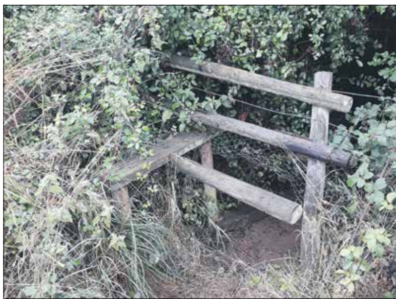
Before work. Photo: Ruth Cornish.
