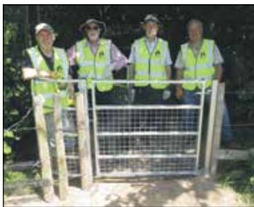
The installation team after installing one of the gates. Left to right: Alan Robinault, David Moffat, Graham Croucher, Keith Hawkins. Photo: Ray Sharp (who project-managed the installation).
