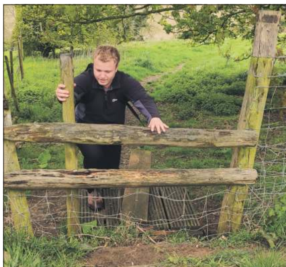
The stile was rotting and difficult to negotiate.
