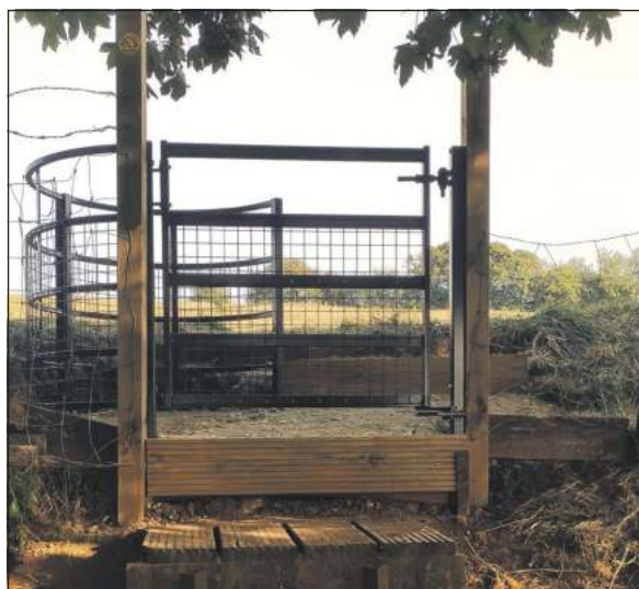
New gate and steps installed by White Cliffs Ramblers.
