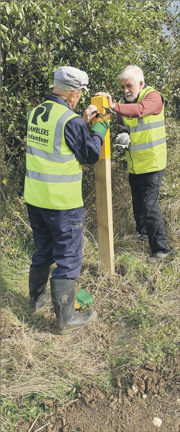
Installing a new yellow-topped marker post.
