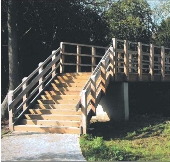
Sherwood Bridge on Studios Walk.
