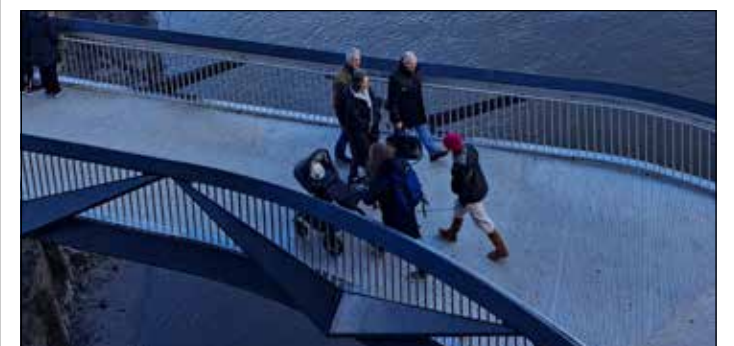
The elegant new footbridge takes walkers under Barnes Bridge.
