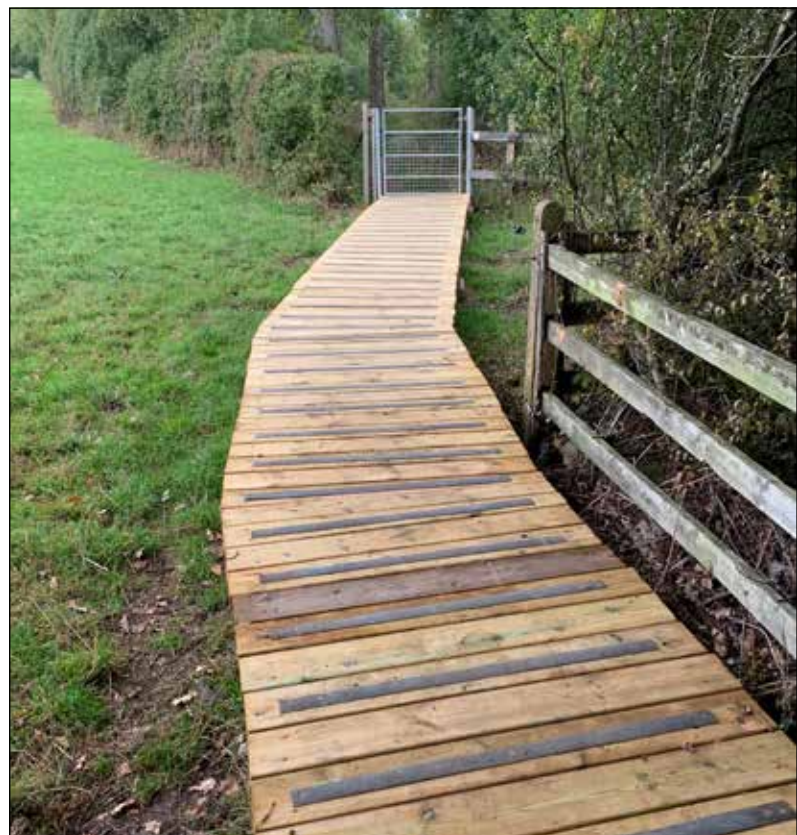
The new boardwalk.
