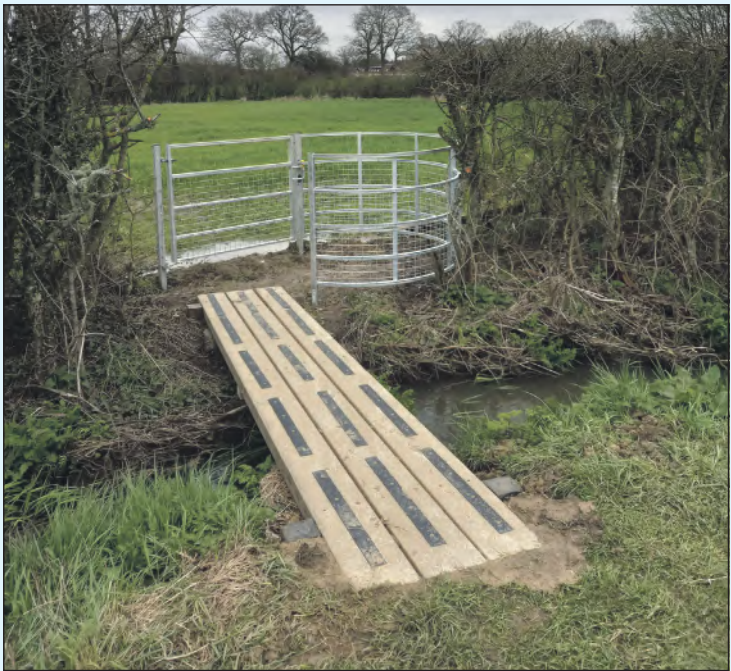
A new footbridge and gate on Footpath 248 off Tandridge Lane. Photo: Barbara Bulman
