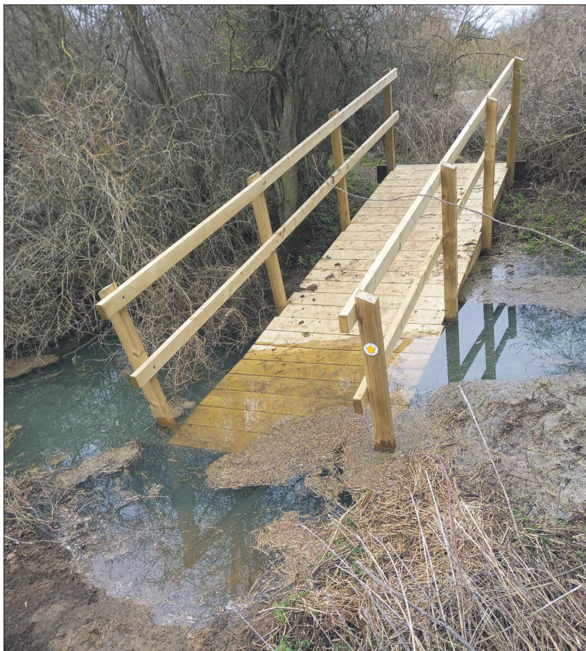
When is a bridge not a bridge? At least it has a waymark disc on it!
