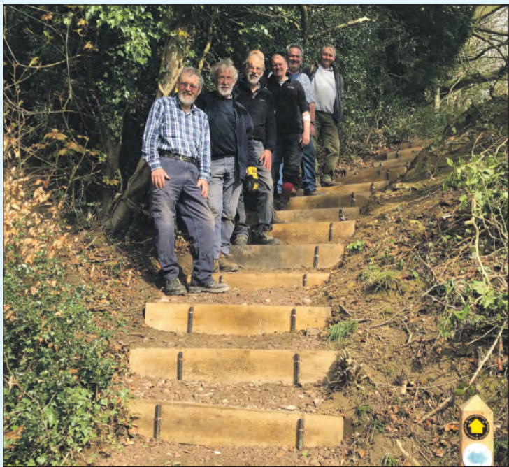
The work party at the new steps.
