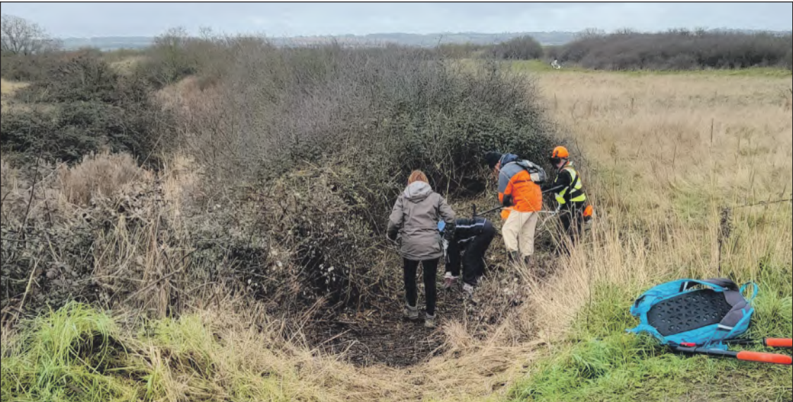
Work begins on the Hullbridge path.
