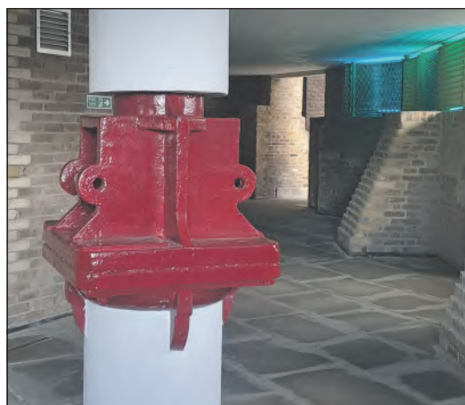
The large metal joint painted in the City's heritage red. Photo: Des Garrahan
