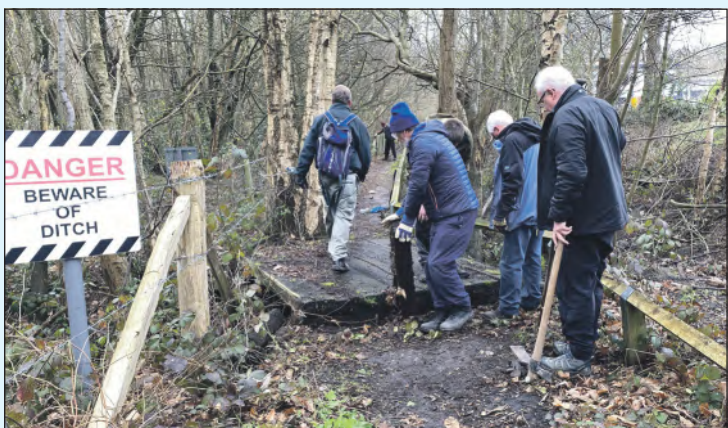
The Guildford footpath team prepares to build a ramp either side of a sleeper bridge. Photo: Brian O'Connell
