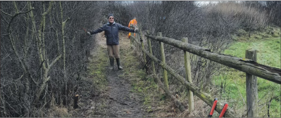
The path restored.
