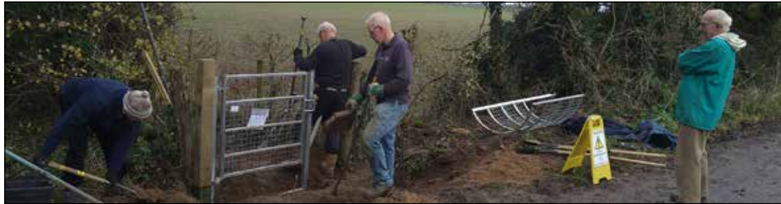
Installing a new kissing gate to replace a stile.
