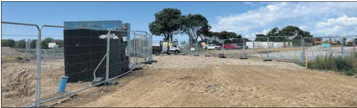
Gates across the North Downs Way at Guston while works take place.
